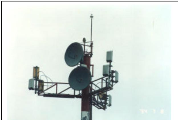
Fig. 9: Cellular phone system antennae installed on horizontal extensions. The antennae face a higher risk of being struck by lightning in this case.
