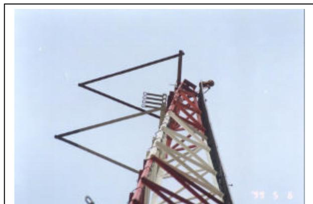
Fig.8: A radio system antennae installed near the top of the mast and protected between two simple triangular shaped horizontal air terminals.
