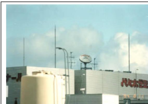
Fig. 12: Three extended Franklin rods being used to provide a wide area of protection for a large satellite antenna and several other antennae.
