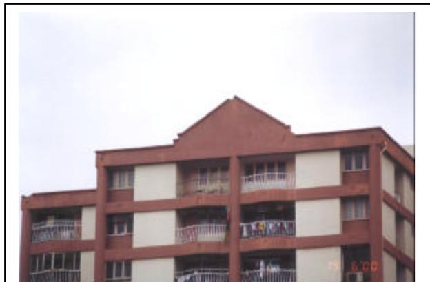
Fig.2: A highrise apartment building showing two typical lightning damaged locations (top of façade and corner on far left).
