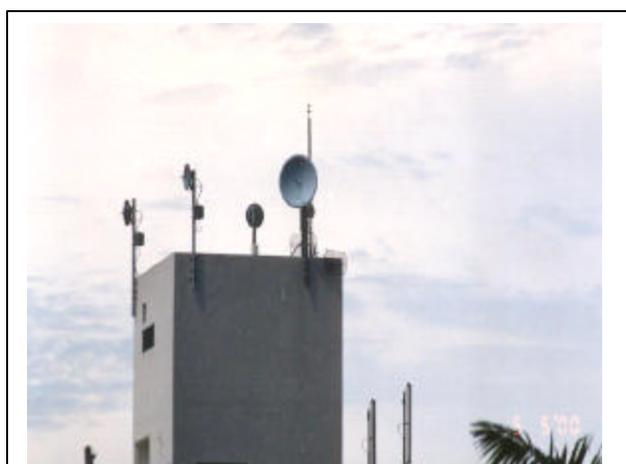
Fig. 6: Several microwave antennae installed on a roof that has been installed with a proprietary lightning air terminal.
