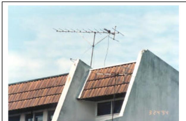
Fig.5: A TV antenna installed close to a PSP, with an already damaged PSP nearby.
