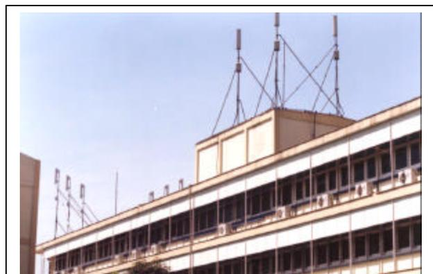
Fig. 7: Cellular phone system antennae installed on and close to the PSP with two proprietary air terminals installed nearby.
