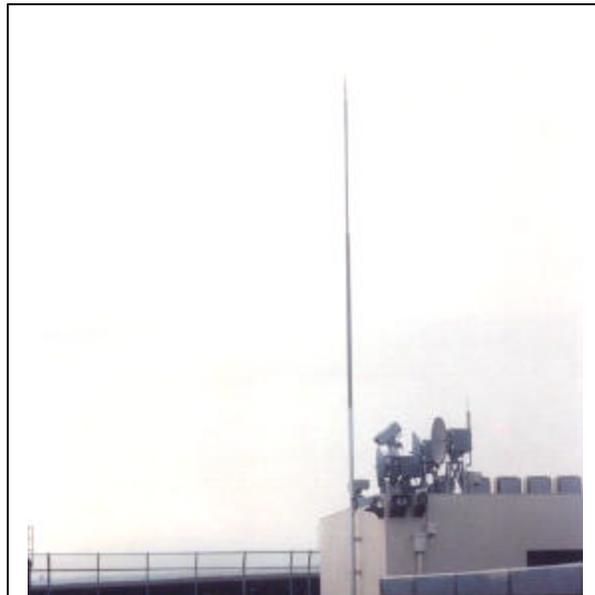
Fig. 10: A single extended Franklin rod used to protect a cluster of antennae on the roof of Narita Airport. The conventional lightning air terminal is widely used in Japan.
