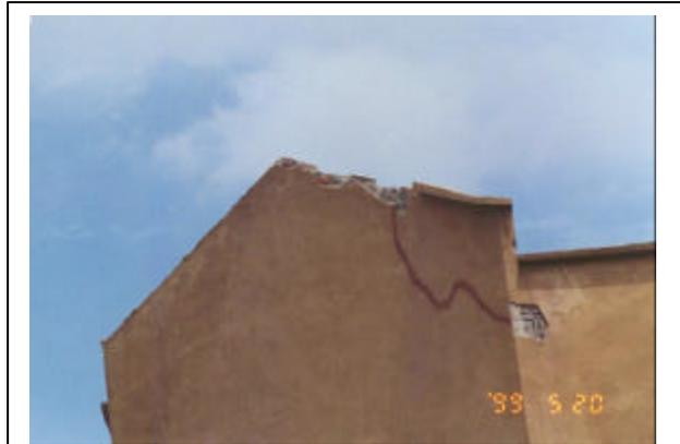
Fig. 1: A lightning damaged façade of a 10m high shop. Several other damaged façades could be found on nearby buildings of similar height.
